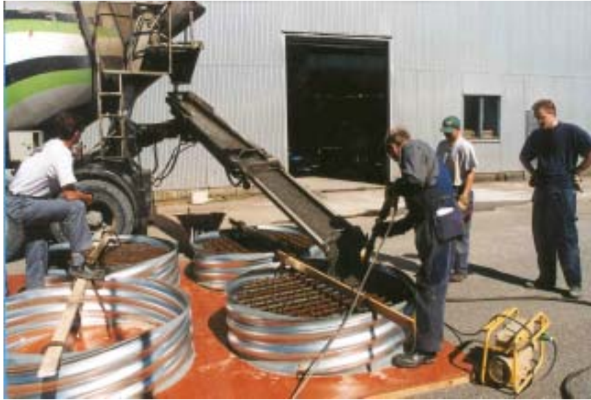
Figure 2.2 Casting of Abetong concrete in June 1999 at FOA, Märsta.
