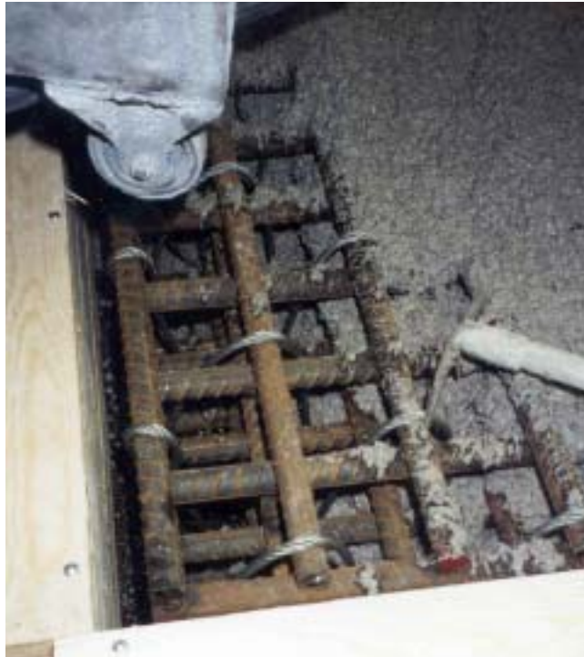
Figure 2.7 Casting of CRC concrete at Densit A/S in February 1997.
