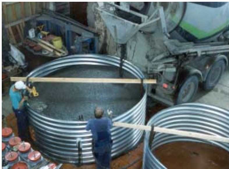
Figure 2.3 Casting of Abetong concrete in July 1999 at FOA, Märsta.
