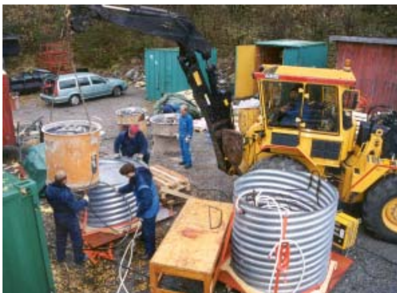
Figure 2.5 Casting of Densit concrete at Vaxholm in November 1997.
