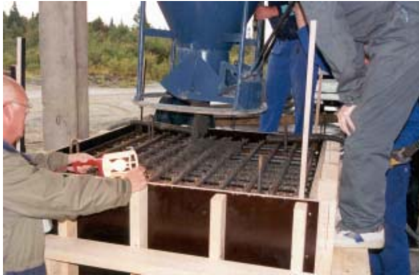
Figure 2.4 Casting of Trondheim concrete in September 1998 in Trondheim, Norway.
