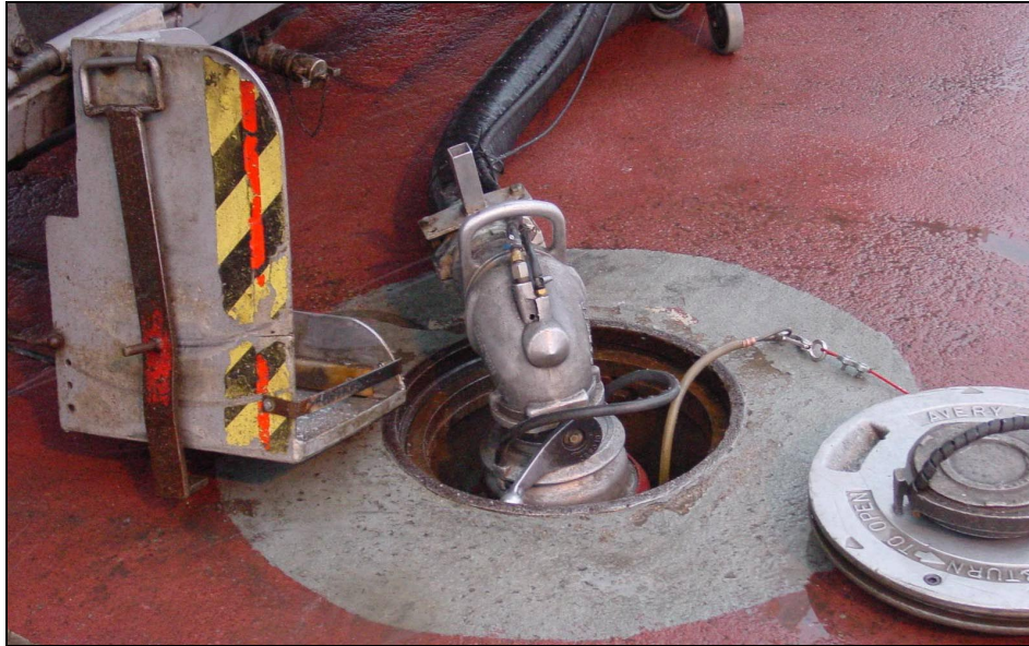
Figure 4-2. A Pit where Fuel is taken for Refuelling. (picture by Bracha, 2002)
